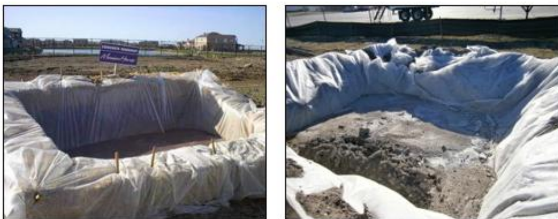
Plate 3-1 Typical concrete wash out areas
