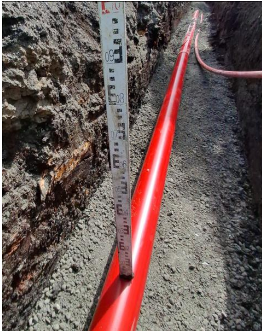
Plate 2-1 Typical Single Cable Trench View
